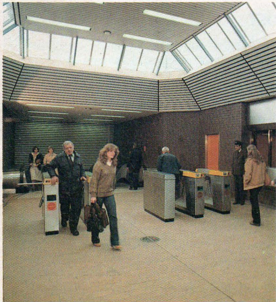
Shields Road underground station
